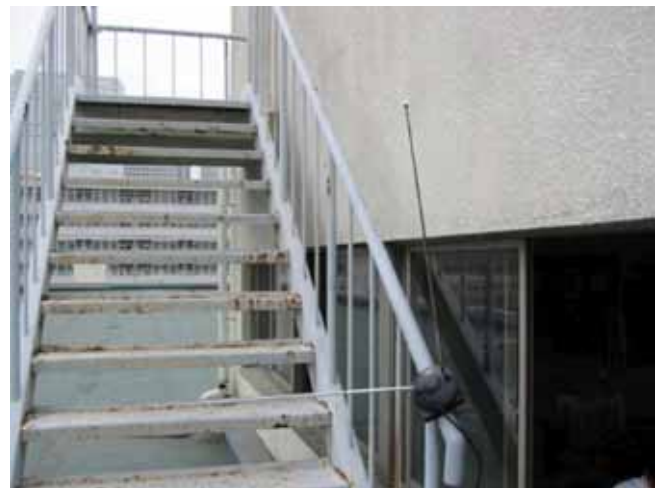
Photo 4 TV Antenna (Rod Type) Settled on the Banister on the Roof of a Five-Storeyed Building in the Tokyo University of Marine Science and Technology in Shinagawa, Tokyo
